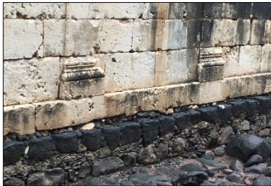
Taken in January, 2018, the black stones are the foundation of the original synagogue existing during time of Jesus.
